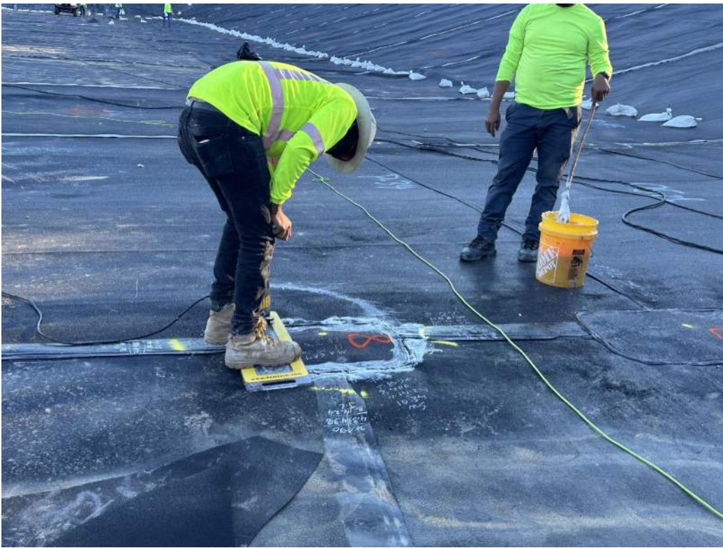
Photo 11 – Geomembrane liner repair testing.
