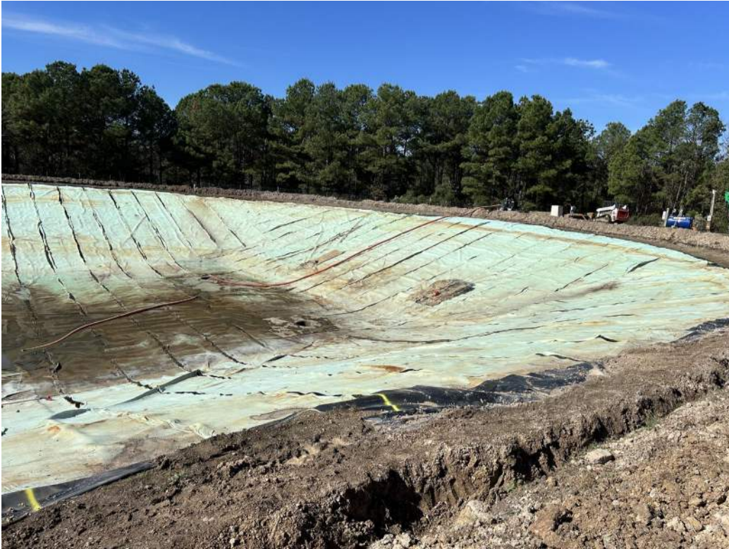
Photo 1 – Existing geocomposite and secondary liner looking northwest.
