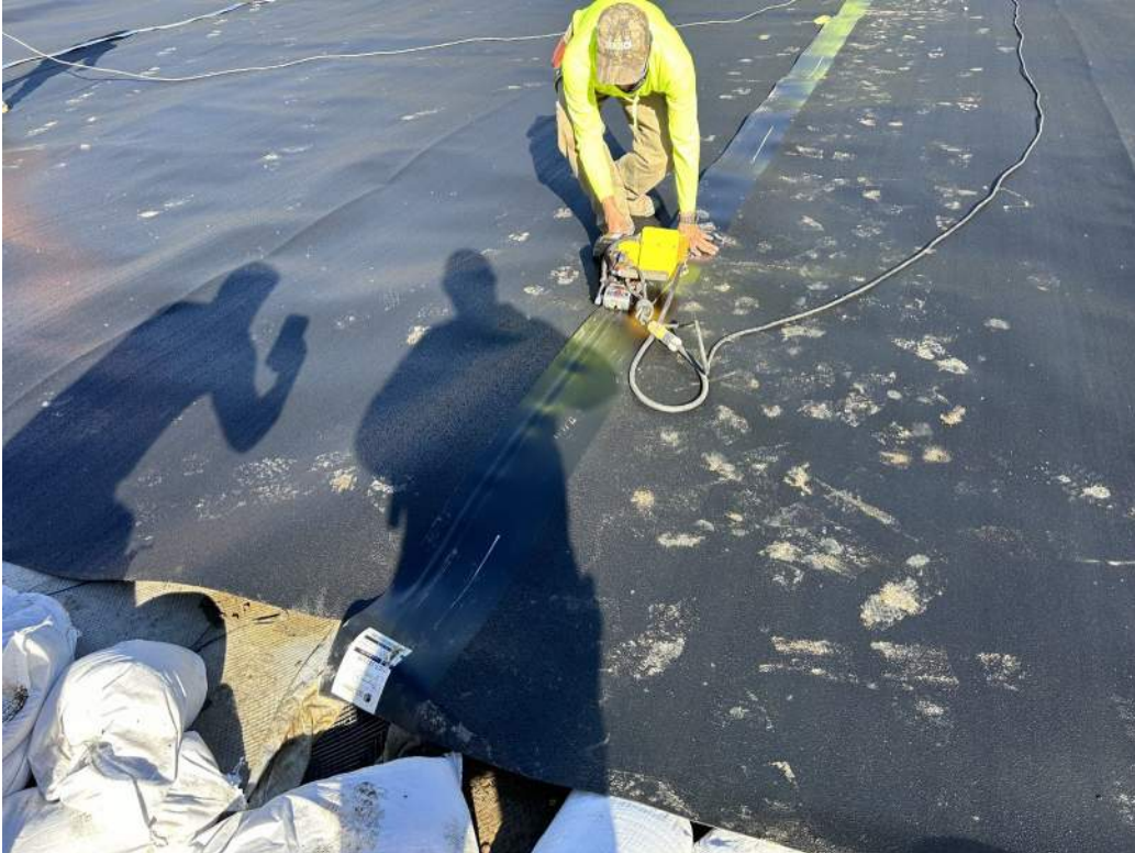
Photo 6 – Fusion seaming of geomembrane liner.
