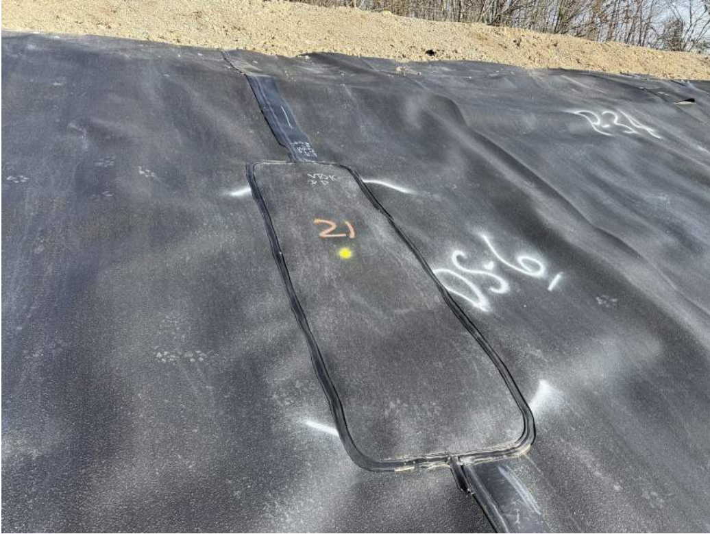
Photo 12 – Typical destructive seam test repair (DS-6).
