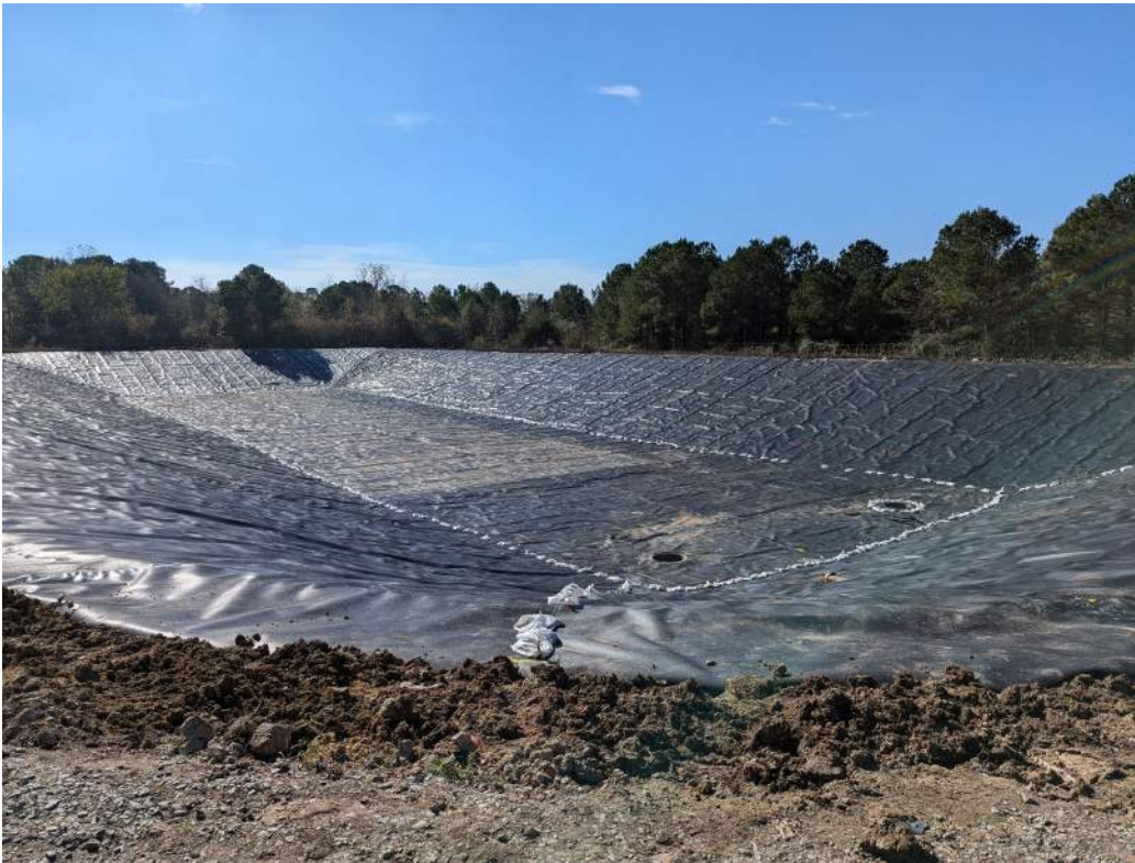
Photo 13 – Completed primary liner installation looking southwest.
