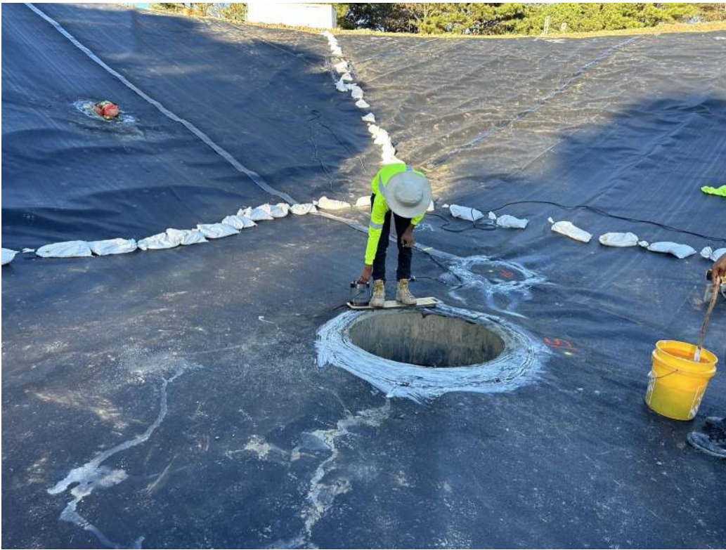
Photo 9 – Seaming and testing of geomembrane liner connection to northwest sump.
