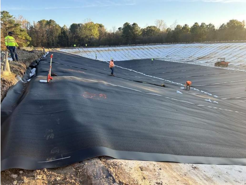
Photo 5 – Deployment of geomembrane over GCL, west slope and bottom.
