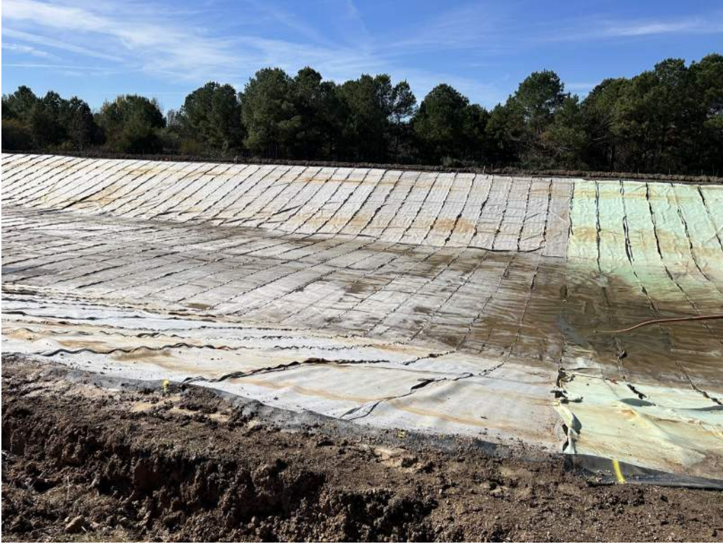
Photo 2 – Existing geocomposite and secondary liner looking west.
