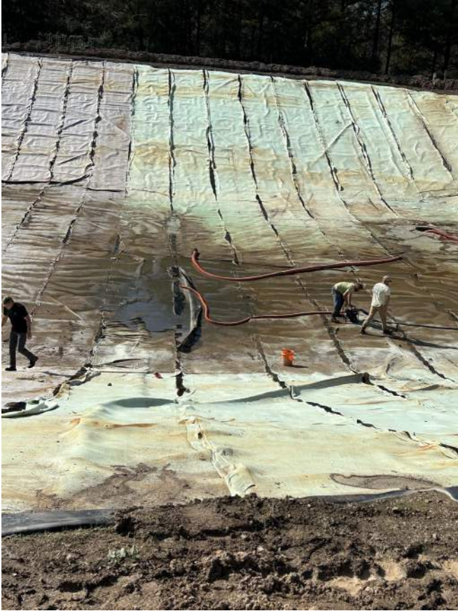
Photo 4 – Existing geocomposite liner preparation.
