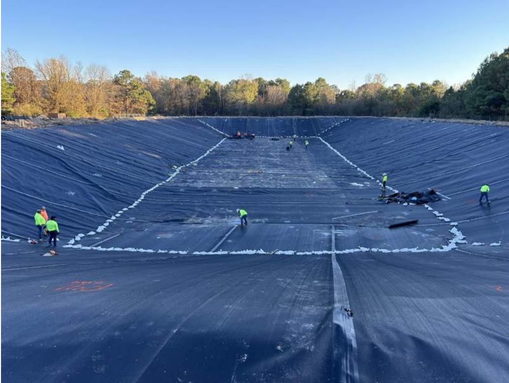
Photo 8 – Geomembrane installation looking north.
