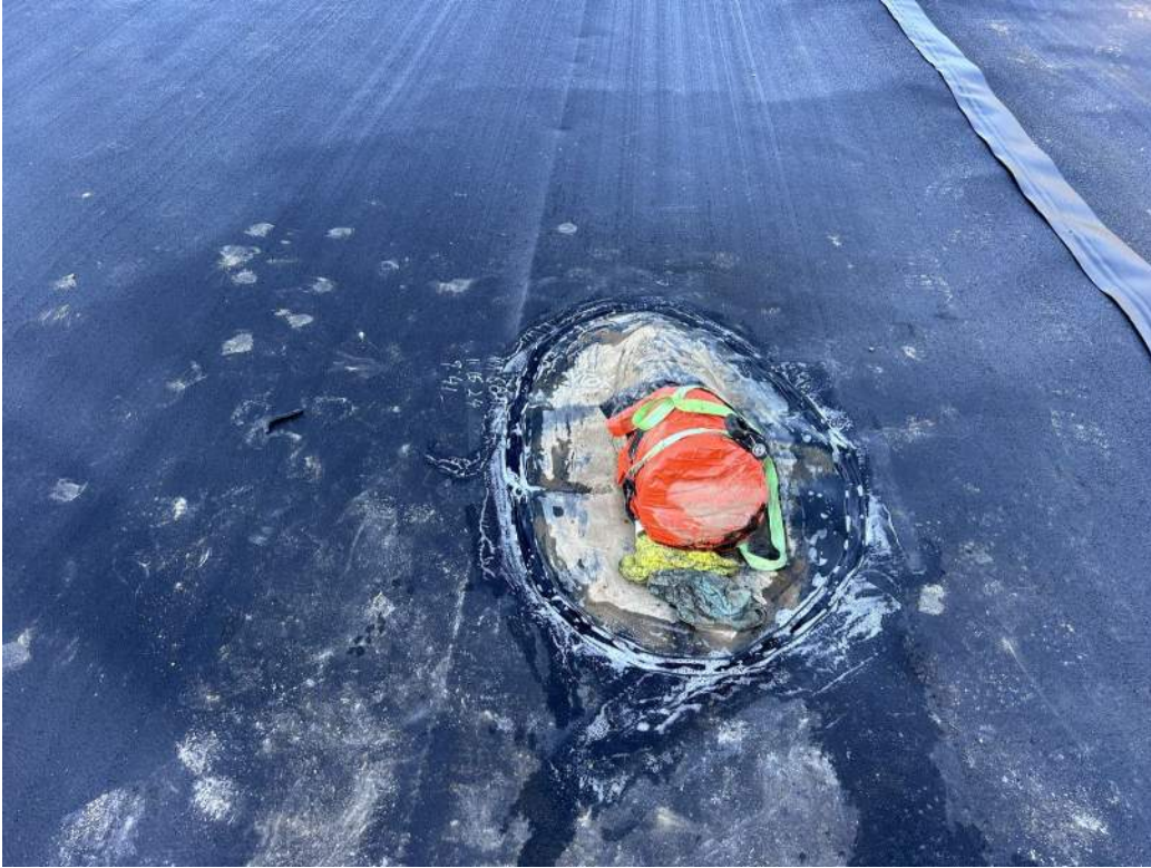
Photo 10 – Typical geomembrane liner pipe boot.
