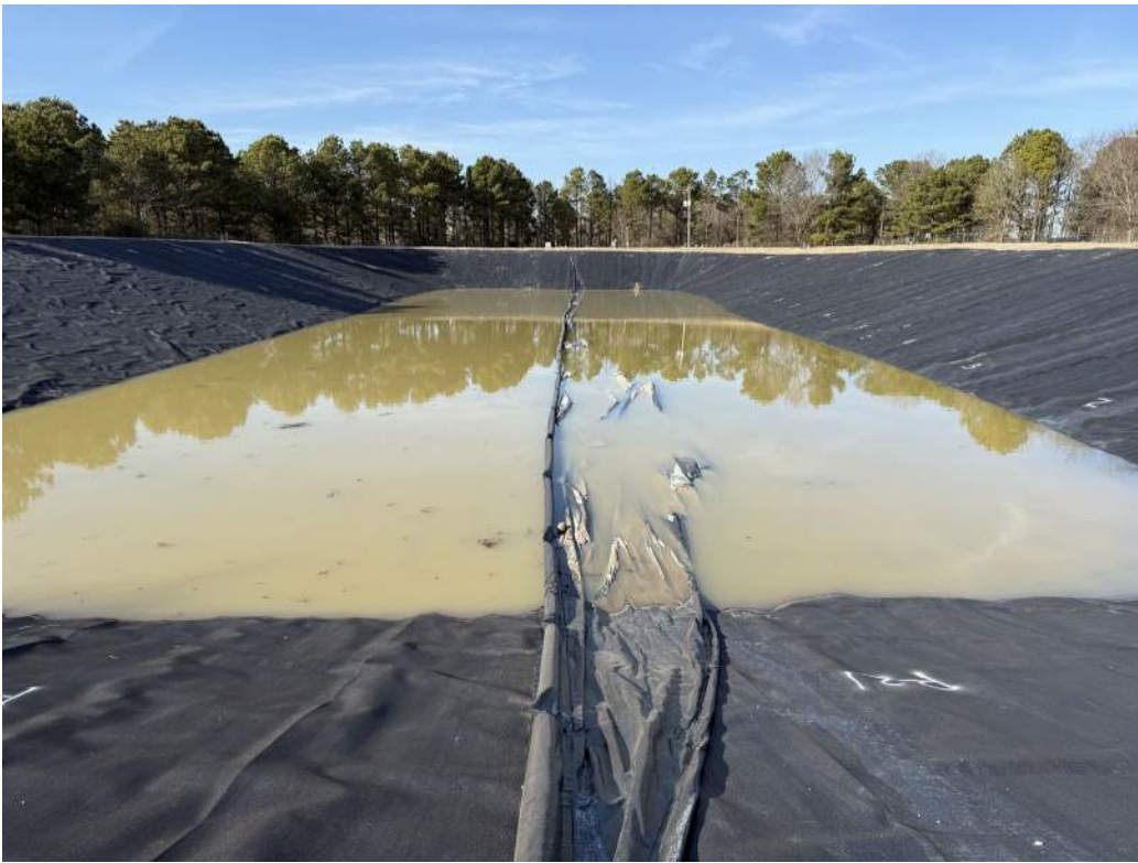
Photo 15 – Pond baffle curtain after installation (stormwater in pond from rainfall).
