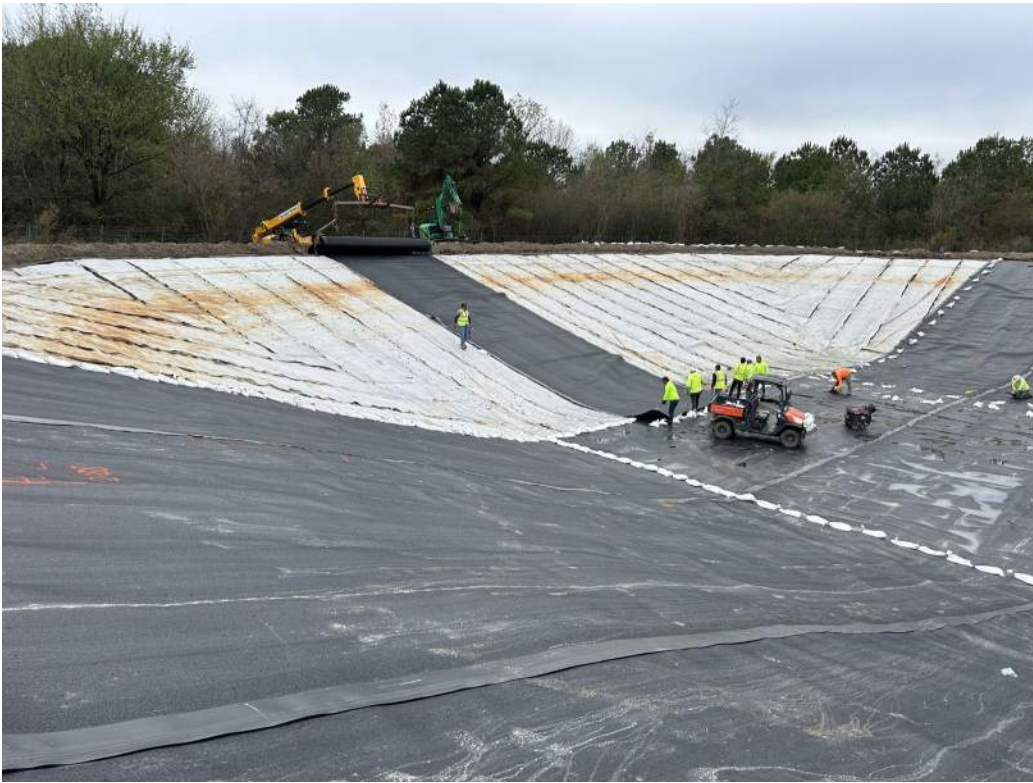
Photo 7 – Geomembrane installation on south slope.
